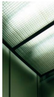
Aluminum Egg Crate or Polycarbonate Diffuser Ceiling Panels
